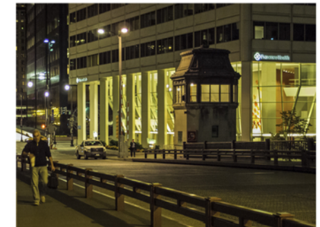
Deck truss at Adams St bridge (Map #16)
