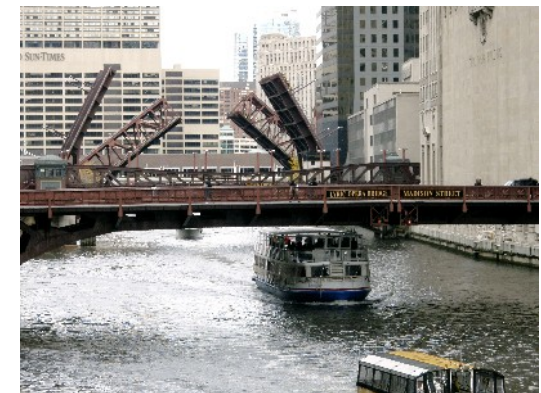
Looking north along the South Branch Chicago River from the W. Madison St. bridge (map #14)
